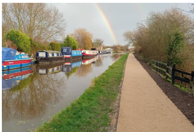
Canal towpath works, Willington
