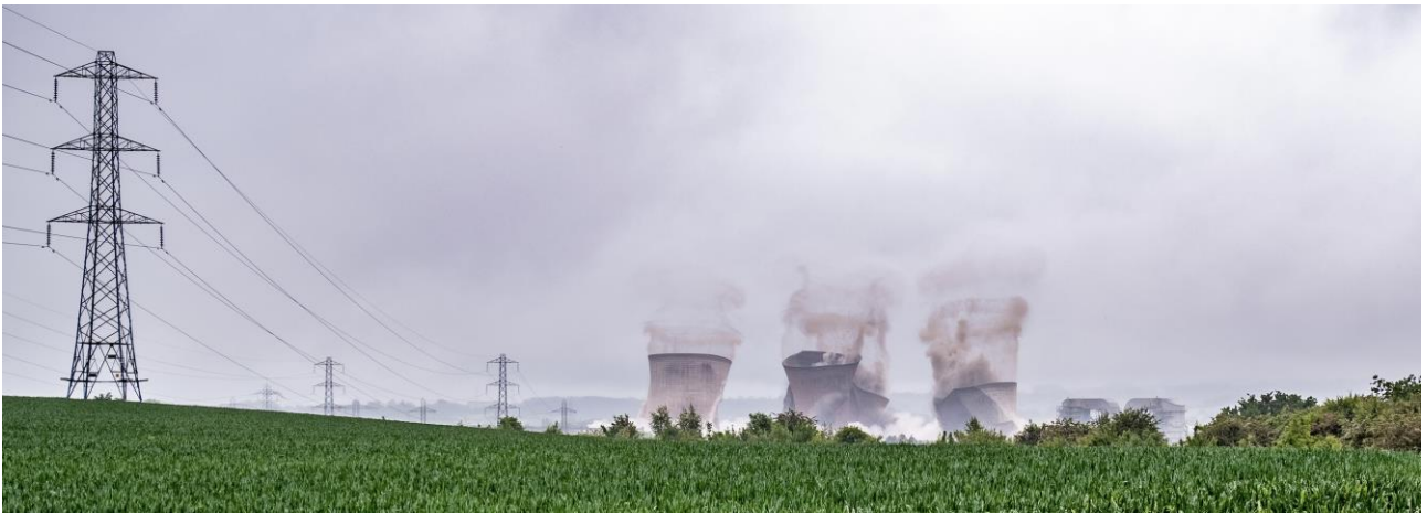
Rugeley cooling tower demolition ~ June 2021. Credit Paul L.G. Morris
