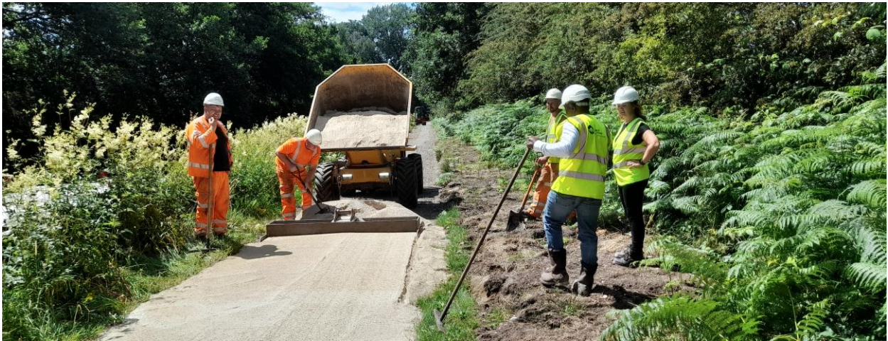
Fradley to Kings Bromley Towpath Upgrade ~ final surfacing
