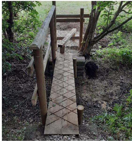
Efflinch bridge ~ before and after access improvements
