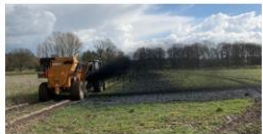
Brook Hollows ~ silt removal, handling and spreading
