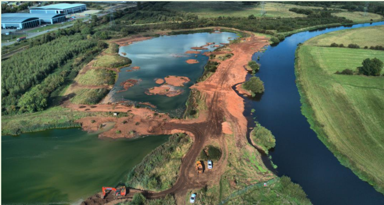
Tucklesholme floodplain reconnection. Credit Jenny France
